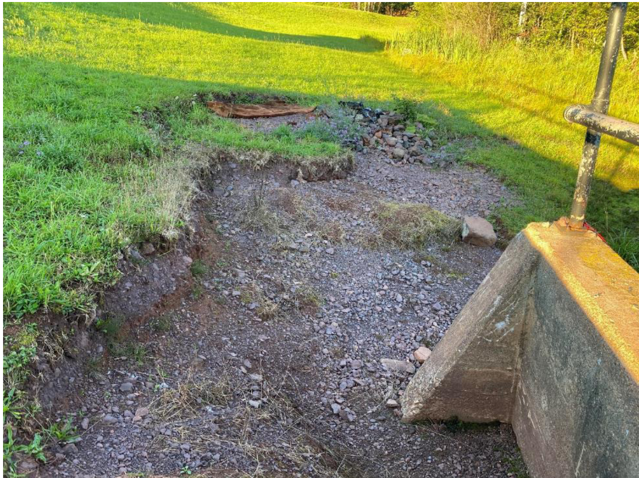
FIGURE 11. AREA OF INTEREST ON THE LEFT EMBANKMENT (WEST WINGWALL) FACING DOWNSTREAM AT THE TOW OF THE EMBANKMENT (August 30, 2022).
