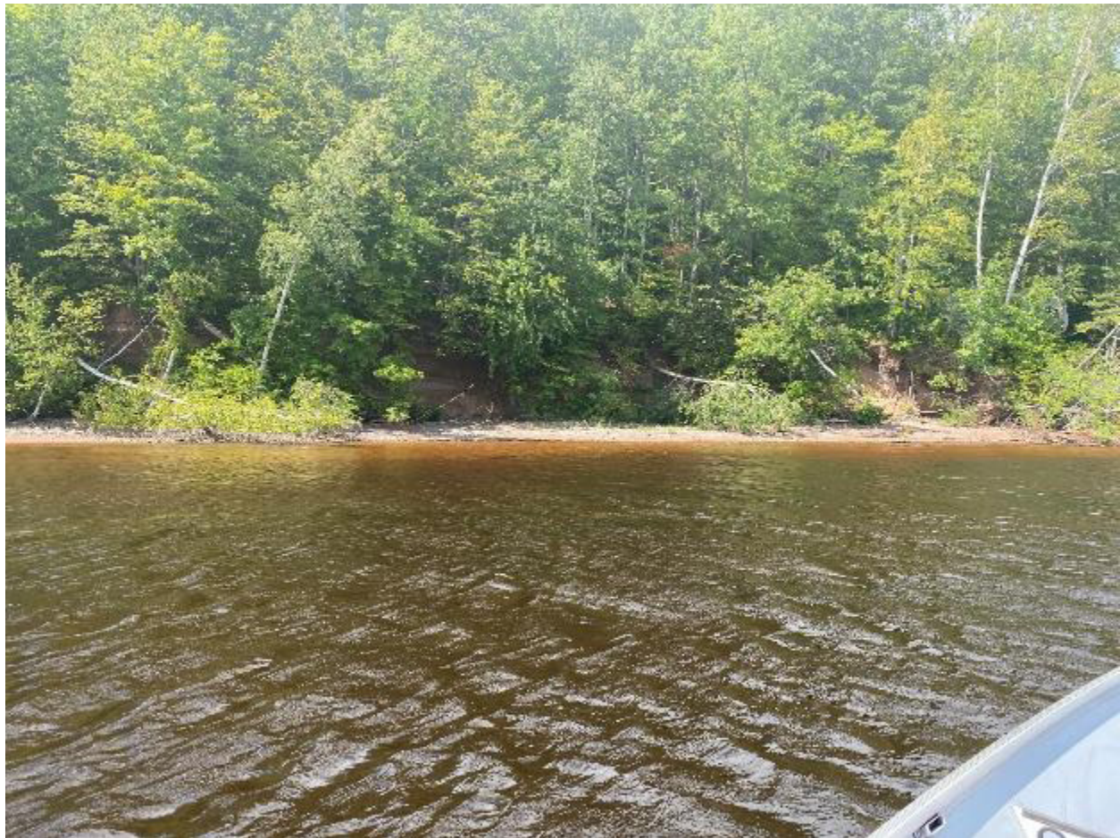
FIGURE 17. SITE #5 FROM THE 2022 GILE FLOWAGE SHORELINE STABILITY ASSESSMENT.
